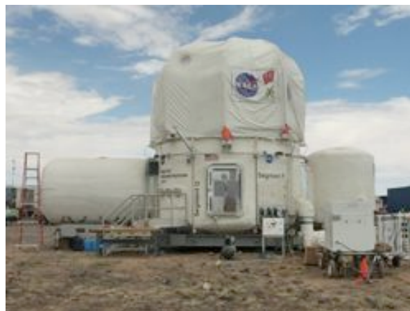
Figure 2. The Deep Space Habitat. The GeoLab antechambers are the 3 circular ports just left of center and the "Segment G" letters.
