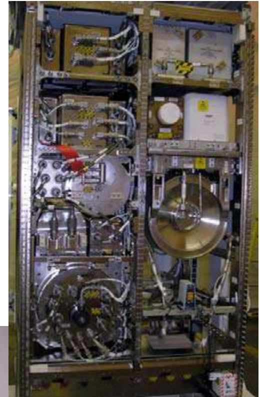
Water Reclamation ISPR Rack
