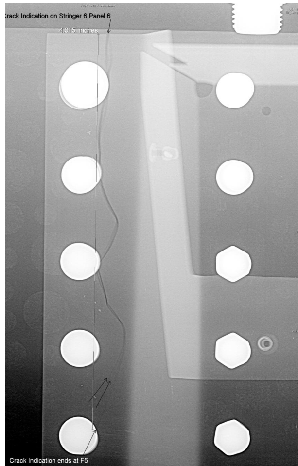
Figure 17. Example stringer crack detected during post-tanking test x-ray inspection.
