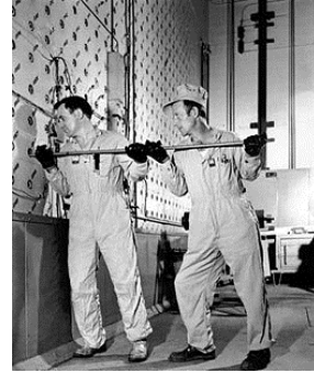
Workers loading fuel at X-10 Reactor
