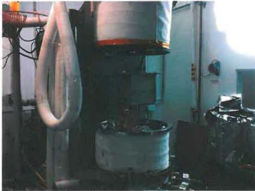
Figure 2-5 Q-Meter Installed, Minus Blanketing
