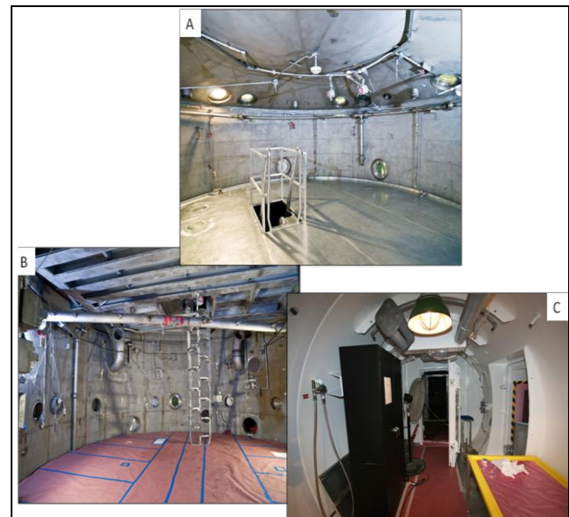
Figure 7: Interior of the 20-foot chamber; A is level 3, B is level 1, and C is the man lock
