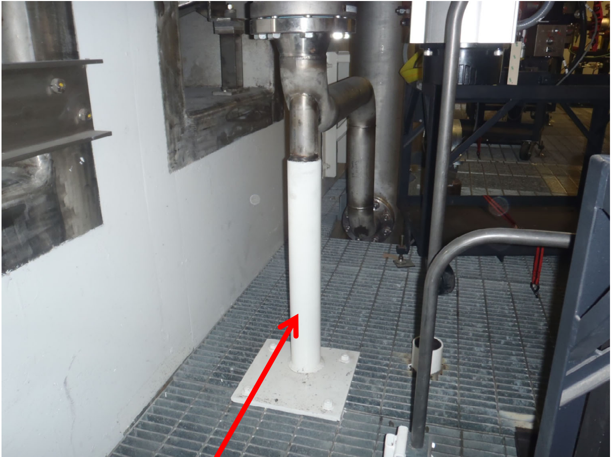
4 inch Riser Elbow Support (PS-8)
