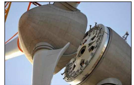
Crane Hoisting Propeller onto Windmill
