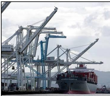
Ship Handling Facilities
