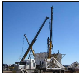
Drilling Rig Assembly
