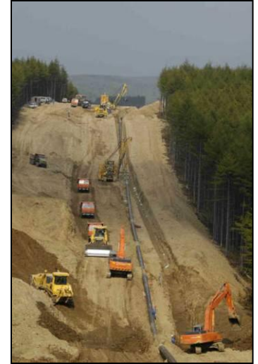
Pipeline Right of Way
