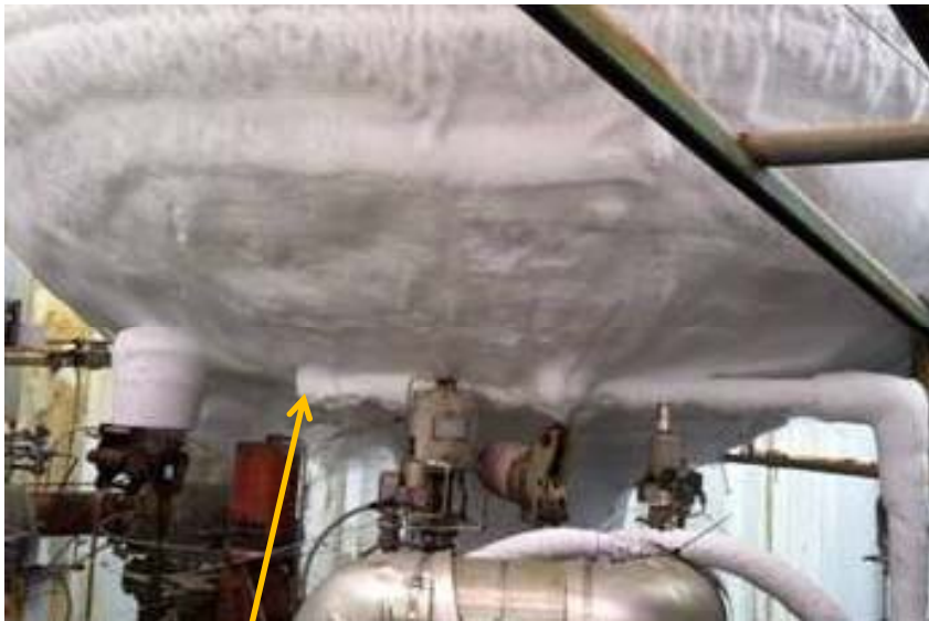
1/4" Instrumentation Port used for Vacuum Service
