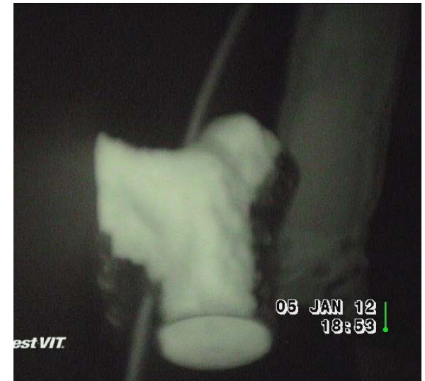
Lower Vacuum Header Disconnected
