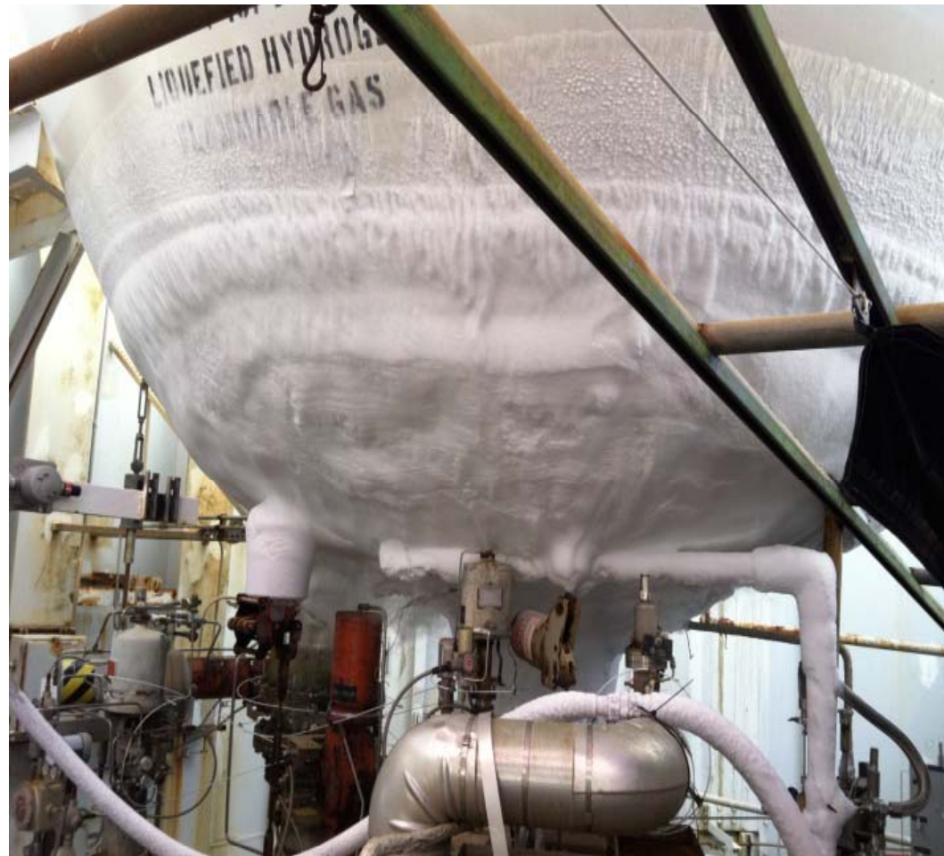
Bottom of LH Run Tank at Low Temperature
