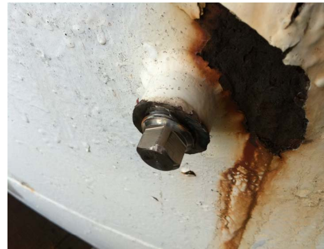
Plug Removed for Vacuum Connection to AE port
