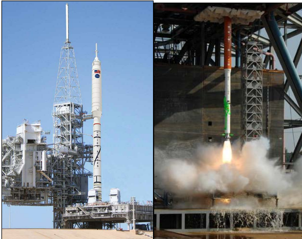
Fig. 1 Ares 1-X on the Mobile Launch Pad (MLP) at Kennedy Space Center Launch Complex 39-B and the ASMAT 5% scale model in a lift-off condition at MSFC ETA TS 116.
