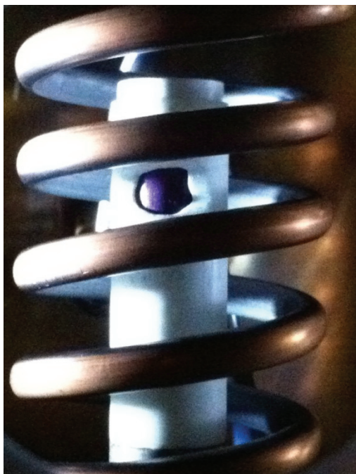
Figure 10. Alumina Insulator installed around fuel element inside 1.875-in.-diam RF coil.
