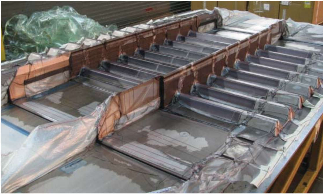
FIGURE 20. COMPLETED RESIN INFUSION OPERATION
