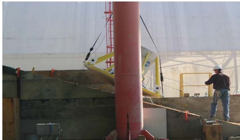
Figure 4. West-side targets on support beams.
