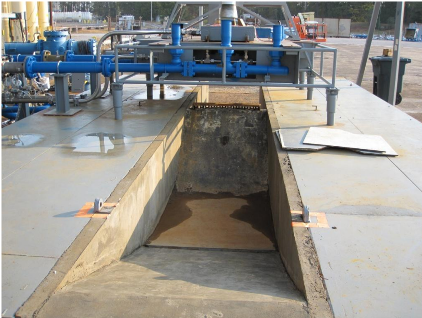
South Side Deflector
