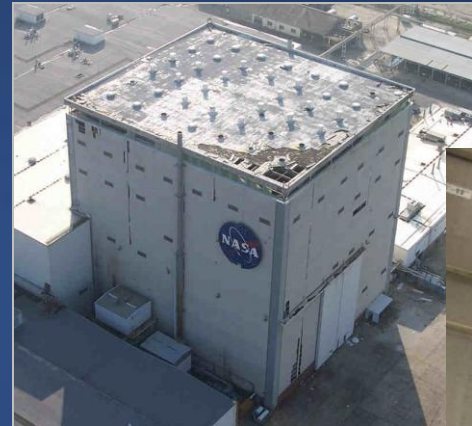
ET-122 Damaged by Hurricane Katrina at MAF
