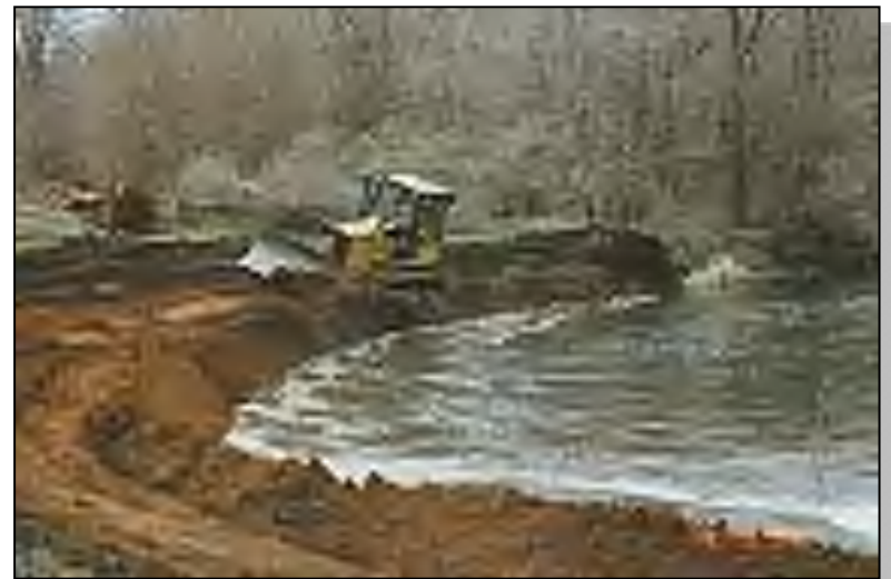
Flood mitigation: Levee construction
