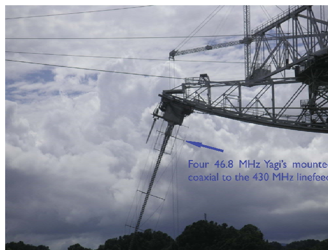
Figure 1. The VHF & UHF antenna feed layout of the AO carriage-house radars.
