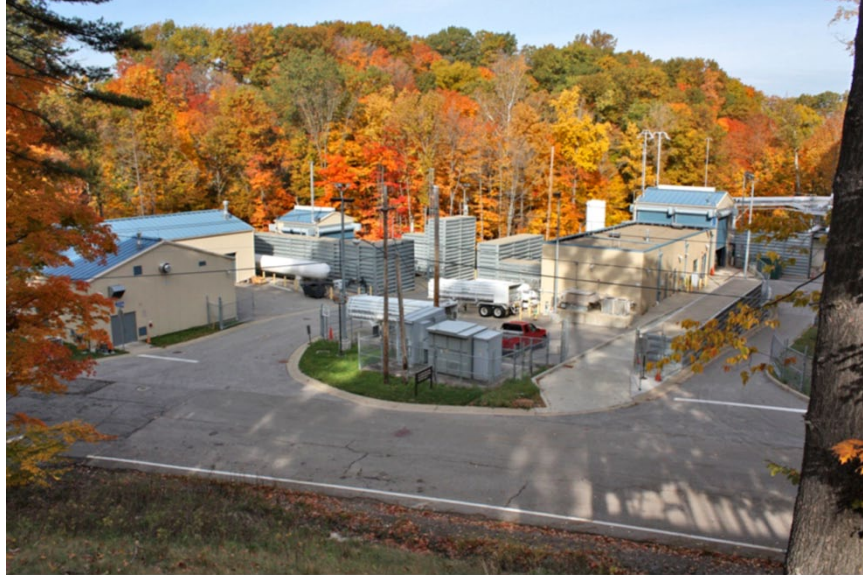
Figure 1.—The Creek Road Cryogenic Complex (CRCC) located at Glenn Research Center.
