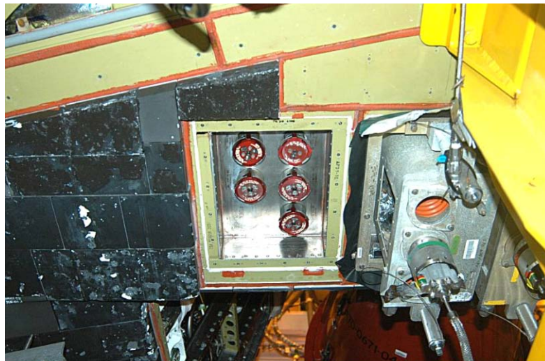
Figure 4-1. Typical Propellant Servicing Opening & GSE Scupper Installation. Fastener receptacles for Door Installation are Inaccessible for R&R
