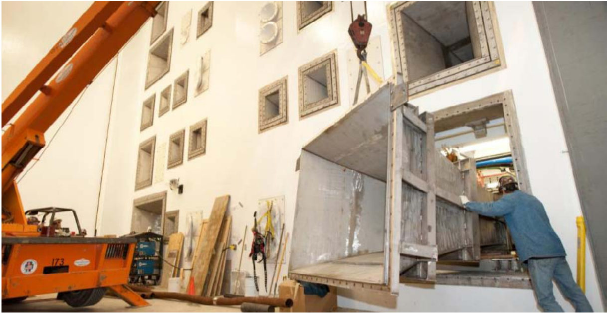
Figure 6.—Construction photo showing the installation of the final RATF horn (25 Hz).
