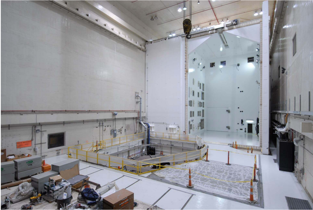
Figure 10.—Construction photo taken November 26, 2010 showing the interior view of the RATF chamber; also visible is the SET mechanical vibration facility (mid-left, below surface level) and the modal test floor (mid-right).
