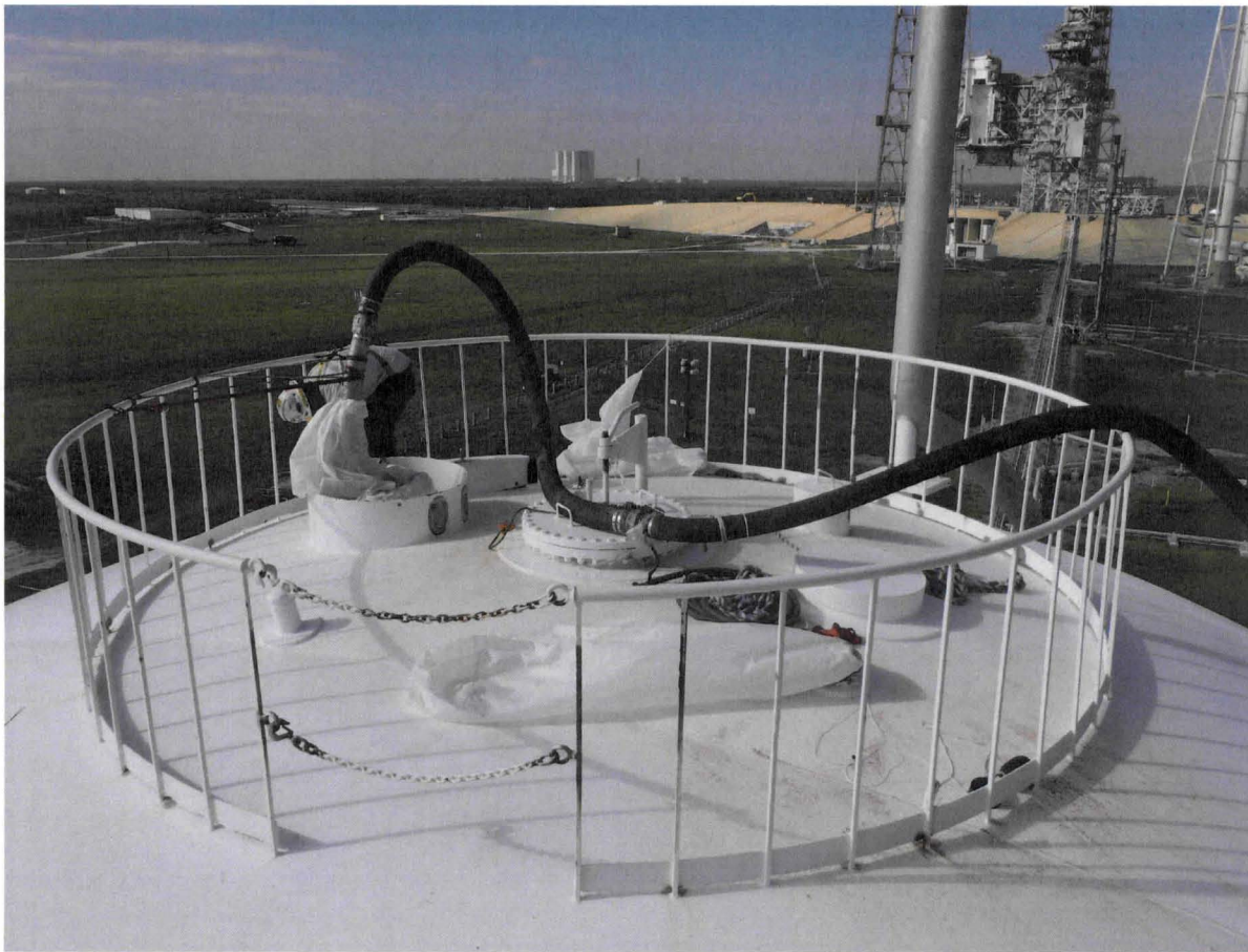
FIGURE 7. Perlite Top-off Fill and Vent Ports
