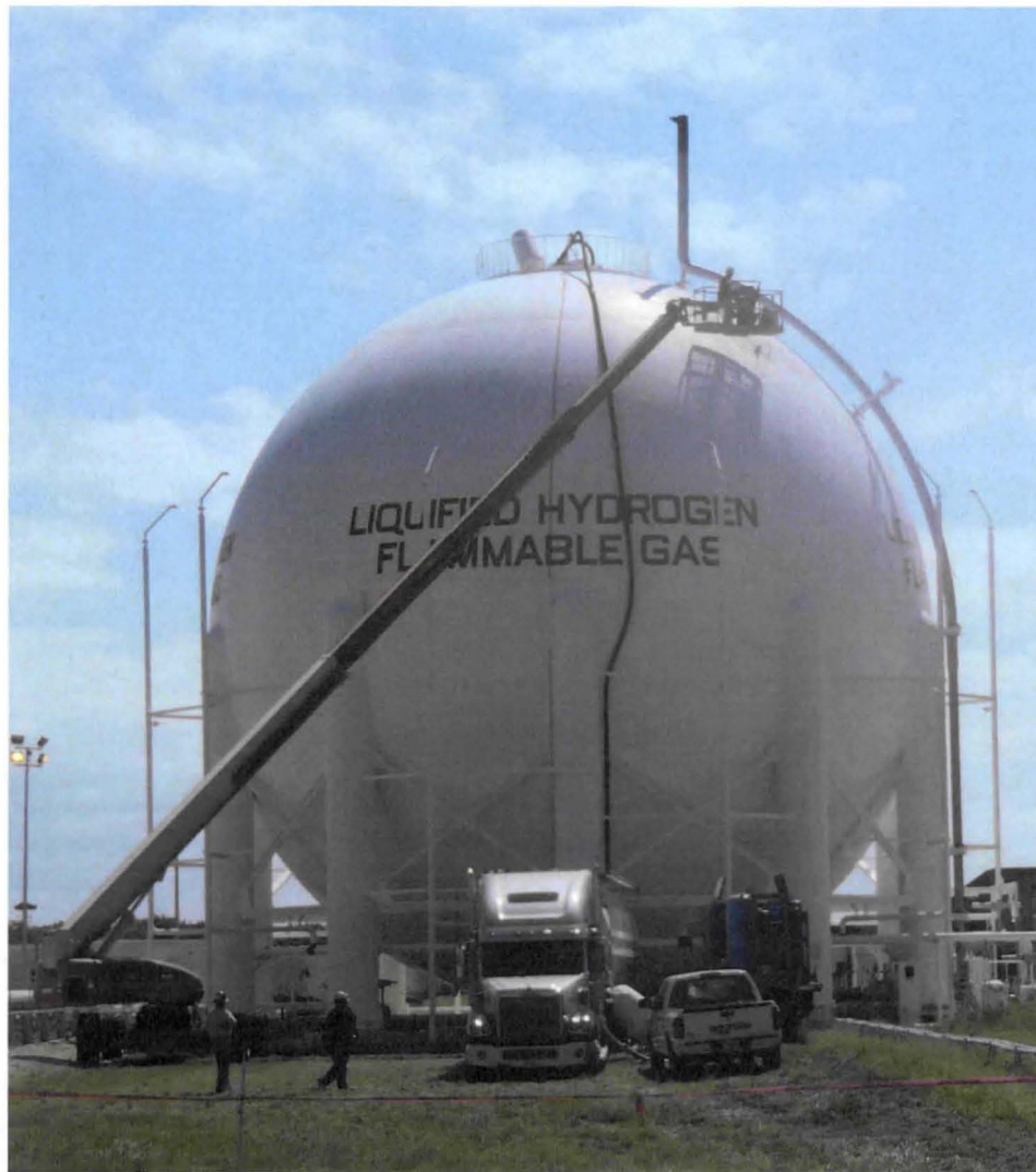
FIGURE 6. Perlite Top-off Set-up
