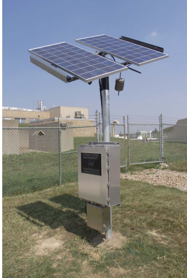
Figure 13.—An ultracapacitor backed photovoltaic power system at GRC.
