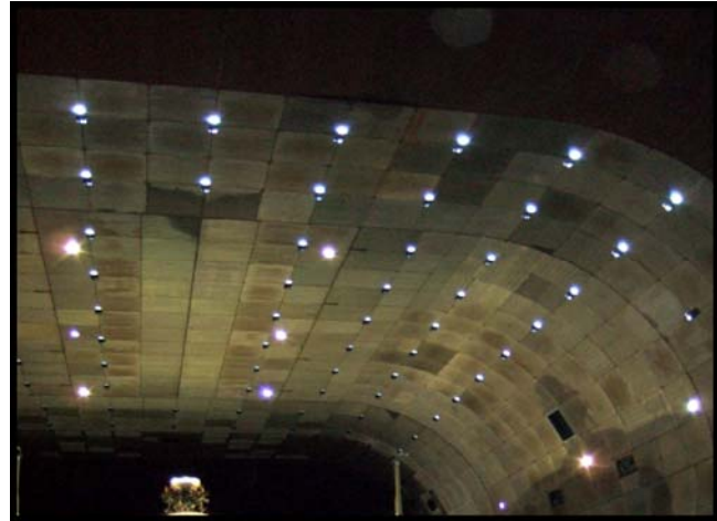
Figure 6. Six-inch diameter retro-reflective calibration targets installed on the test section ceiling.
