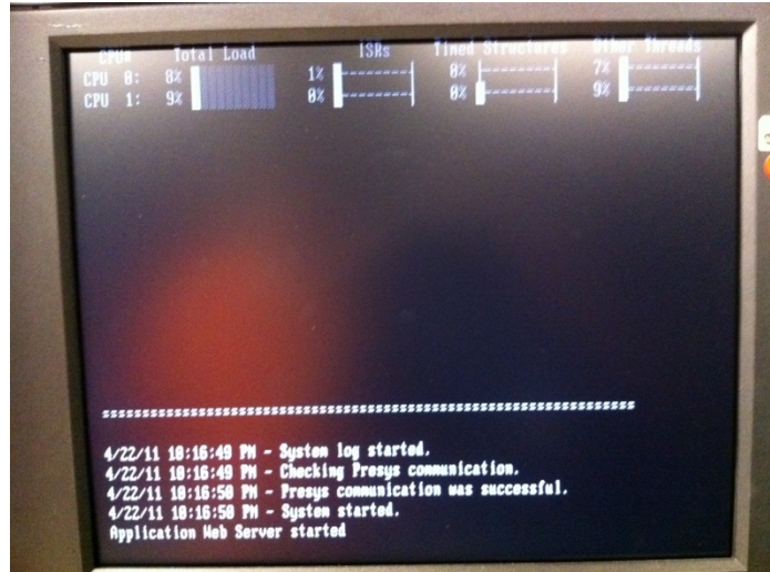
Figure 8, DAS NXLT Command Line Interface
