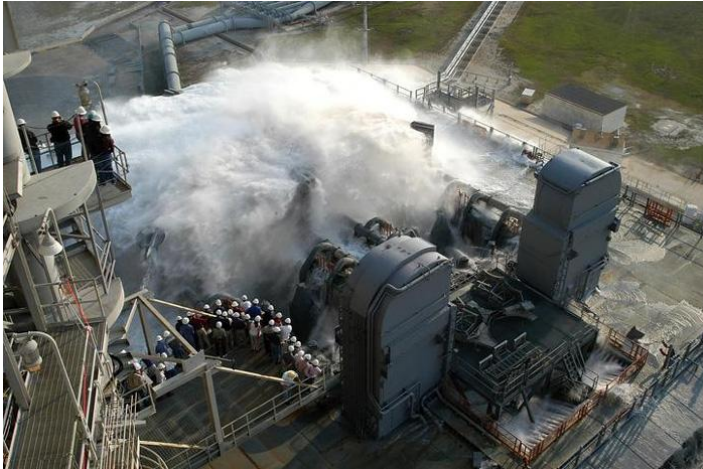
Figure 5-5. Water Spray System and MLP Water Troughs
