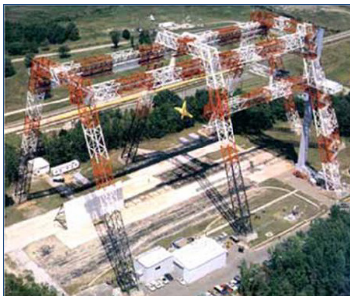
Figure 8.1-1: Photograph of the IDRF Located at NASA Langley Research Center
