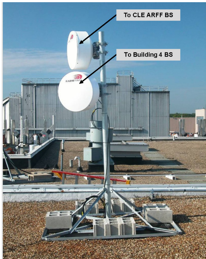
Figure 16.—11-GHz backhaul radio outdoor unites (ODUs) at NASA Glenn Building 110 with links to NASA Glenn Building 4 base station (BS) and to Cleveland Hopkins International Airport’s (CLE) Airport Rescue and Firefighting (ARFF) building.
