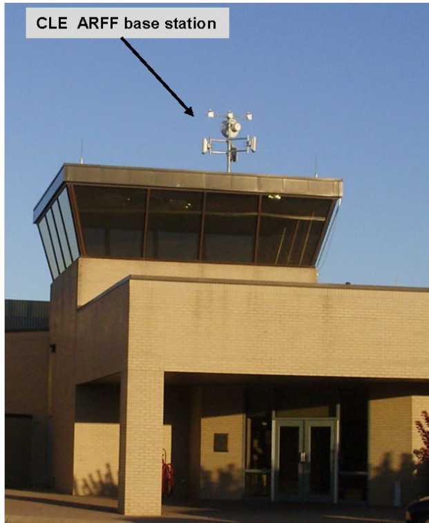
Figure 17.—Aircraft Rescue and Firefighting (ARFF) building base station on observation deck roof.
