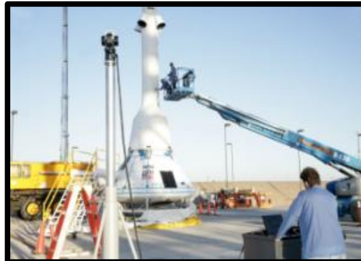
Measuring Stack Straightness with Laser Scans
