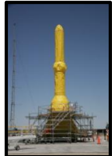
Thermal Cover installed 20
