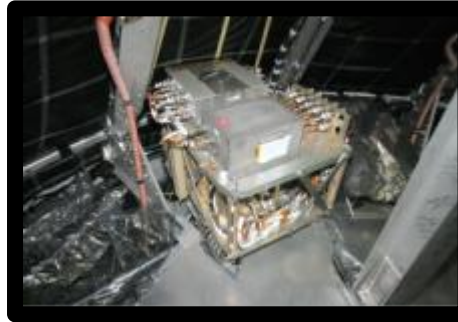
Avionics Pallets and Harnesses Installed
