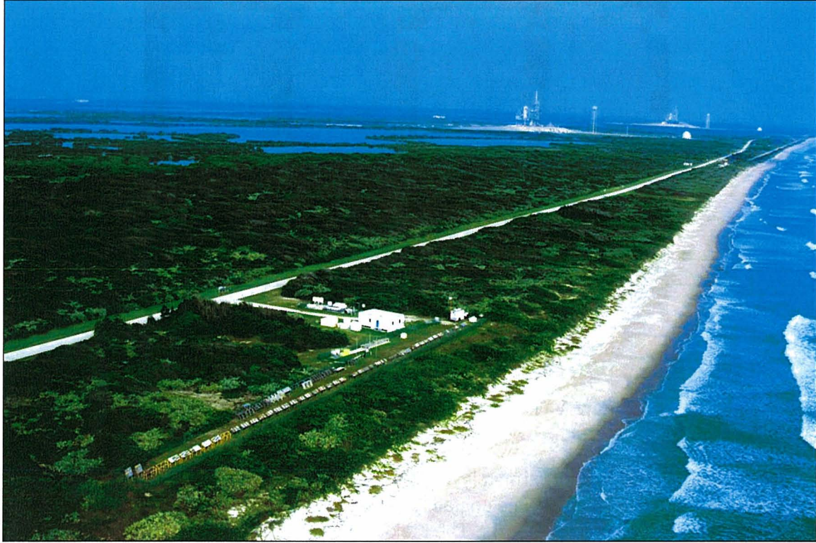
Figure 2. KSC Beach Corrosion Test Site
