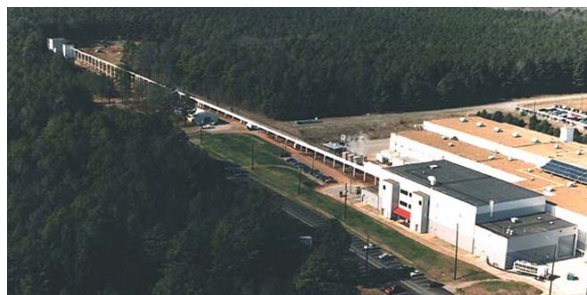
FIGURE 6. The 525m-long X-ray Calibration facility at MSFC. The building to the far left houses the various x-ray sources and filters. The building to the far right houses the large thermal vacuum chamber that held the telescope and various detectors during x-ray calibration.
