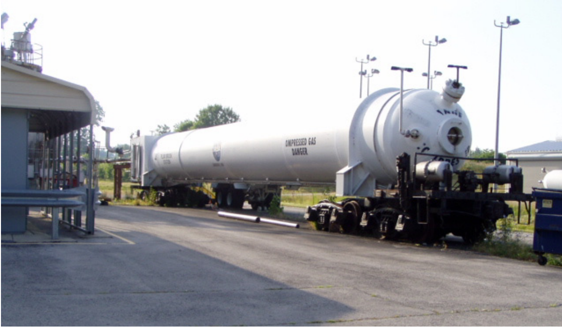
Figure 3.—HTF facility railcar providing gaseous nitrogen supply.
