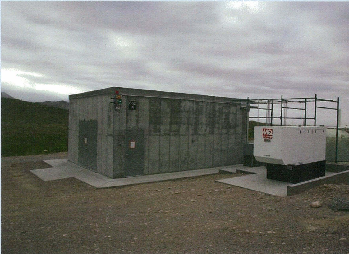
WSTF Test Cell, thermally controlled test cell with generator back-up. Precludes thermal control concerns akin to those of the LLNL tests.
