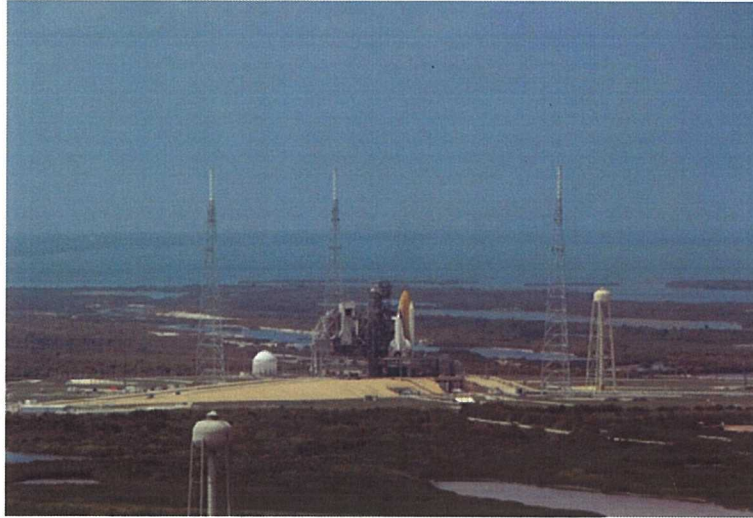
Figure 1. New lightning protection system at Launch Complex 39B, at the Kennedy Space Center, Florida.
