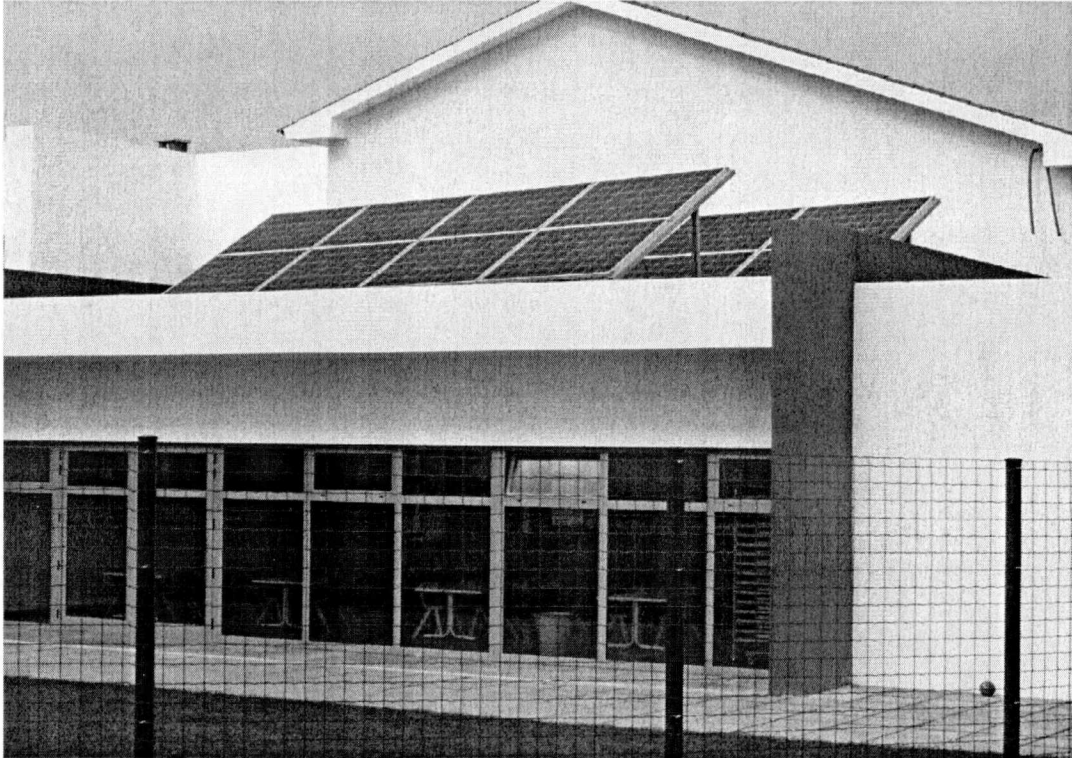
Solar panels at Santa Cruz Public High School, Torres Vedras, Portugal
