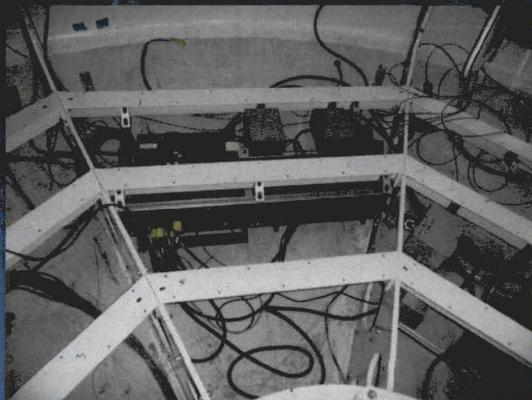
120 VAC PDUs, 120VDC and 28VDC Power Supplies in Sub-Floor
