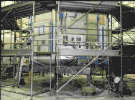
HDU Prepared for Insulation Application
