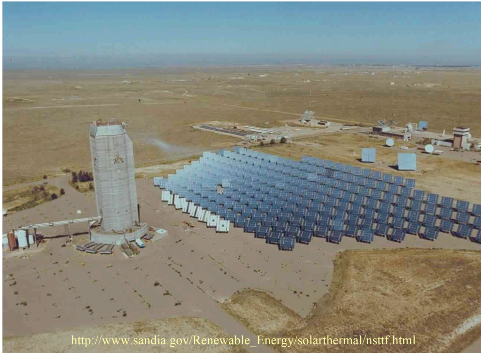
Figure 2. The Solar Power Tower uses an array of heliostat mirrors to focus solar radiation on the test target located at the top of the tower or the wind tunnel test bay.
