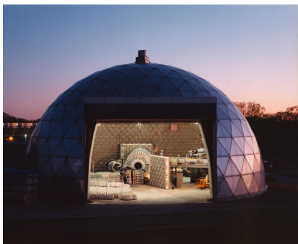
Figure 1.—Aero-Acoustic Propulsion Laboratory.
