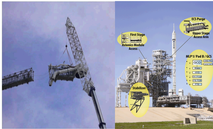
Figure 9. Gaseous oxygen arm being removed (left) and artist’s concept (right) depicting hardware added to LC 39B for Ares I-X.
