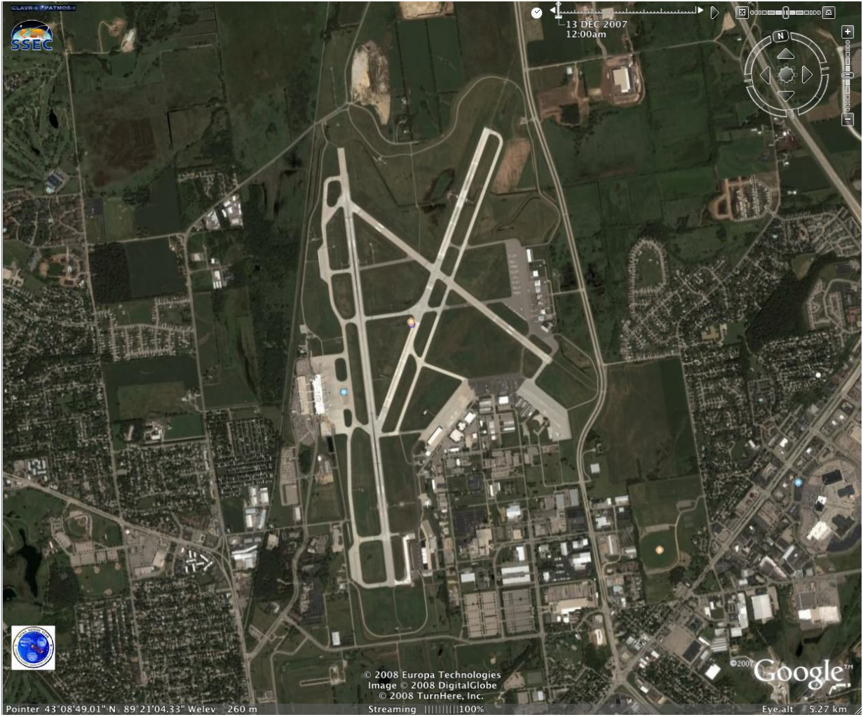
Figure 206. Google Earth Image of Truax Field.
