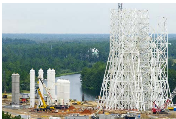
Figure 48. Test Stand A-3 under Construction at SSC
