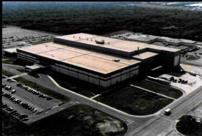
Space Station Processing Facility
