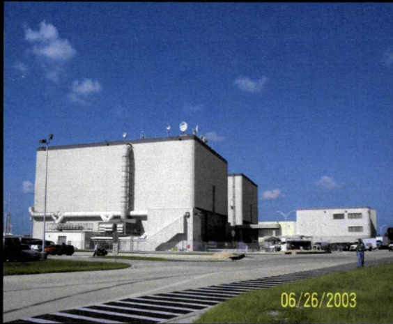
Orbital Processing Facility
