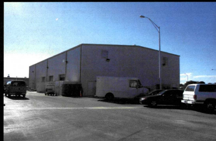
Payload Maintenance Facility
