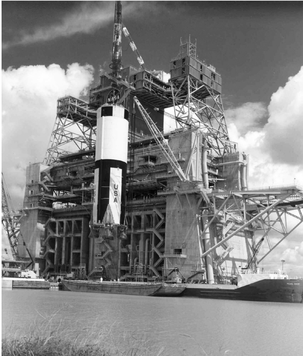
S-1C Stage Installation into Hot Fire Stand at Mississippi Test Facility (MTF) - 1967
