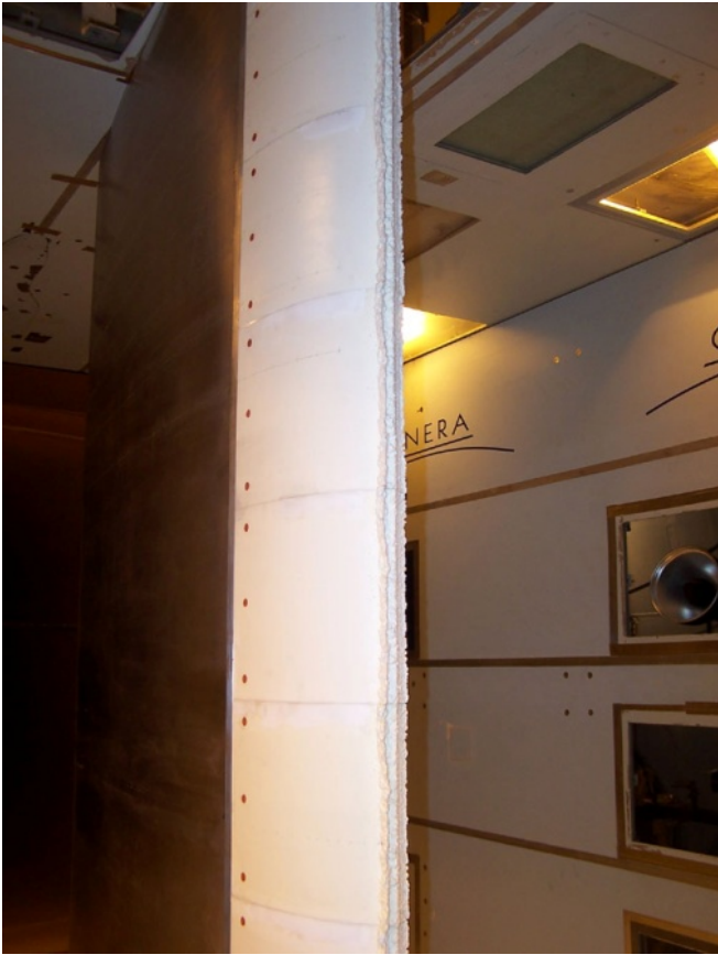
Figure 8.—Completed installation of horn shape EG1164 casting sections on the leading edge of the NACA 23012 airfoil model (upper-surface view).
