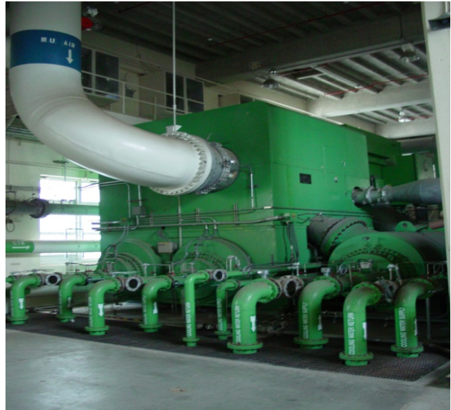
Figure 1. MHI Make up air compressor, out of service.
