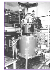
Spin test in NASA Dynamic Spin Rig
