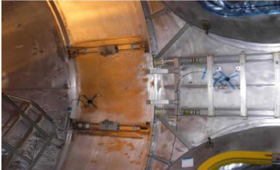
Figure 7.2-2. Photograph of Two DIDS Modules Attached to the Node 1 STA Module Wall
