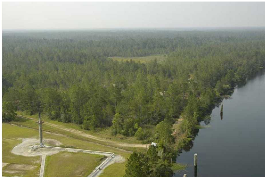
Figure 7 – A view of the SSC A3 test site in May 2007 before construction began
