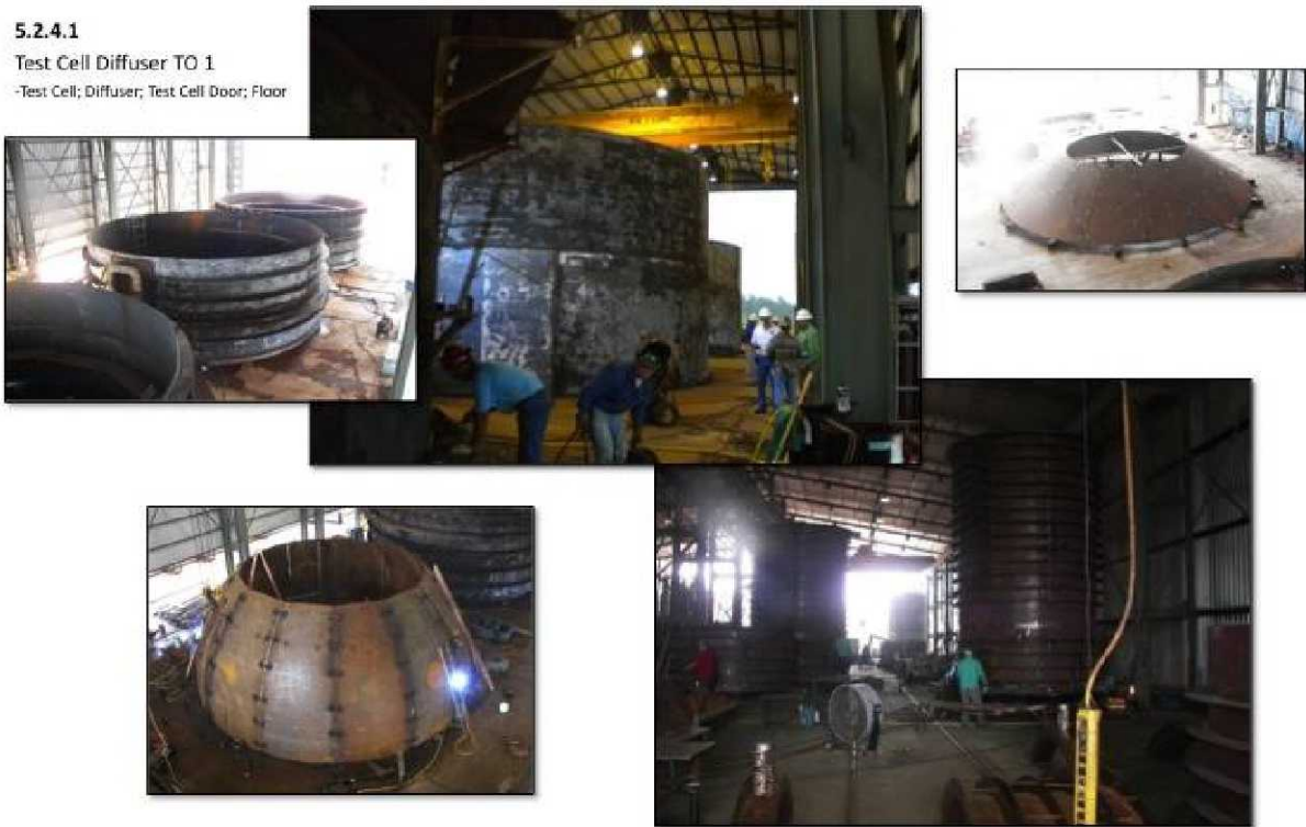
Figure 9 – Photos showing A3 diffuser test cell, floor, and dome in fabrication
