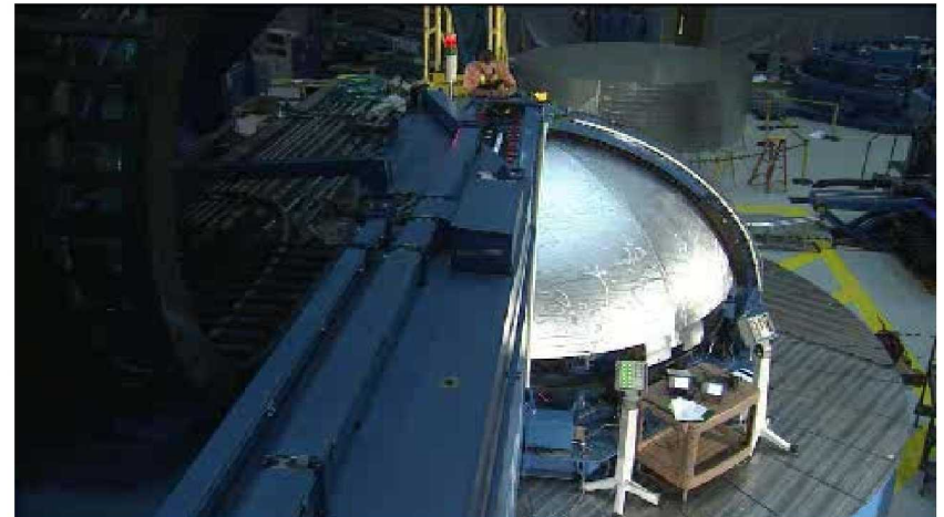
Dome Gore Welding
