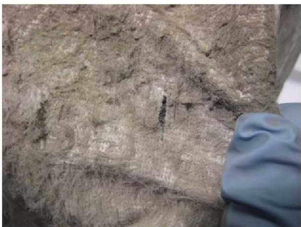
Figure 8. Close-up of damaged Tyvek cylinder. The figure above provides a close-up look at the damaged Tyvek cylinder, including a tear in the fabric.
