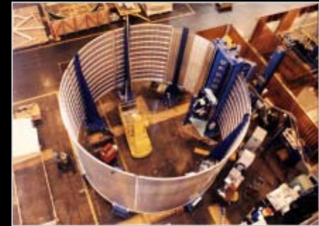
1998 – Welding Shuttle External Tank (ET) Barrel (TRL 6)
